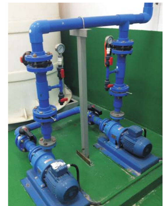
C MAG-PL80 applied for truck unloading of H 2 SO 4 at 96% concentration
