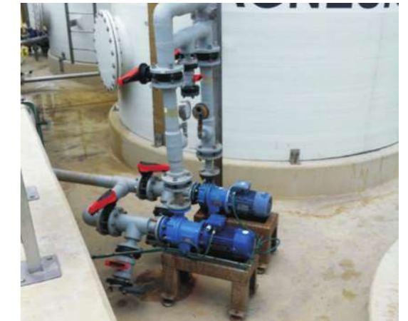
Transfer of Hydrofluoric Acid, Nitric Acid and Phosphoric Acid in a Germany based Fine Chemical Plant
