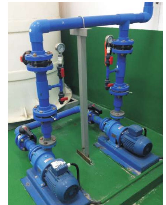
C MAG-PL80 applied for truck unloading of H 2 SO 4 at 96% concentration
