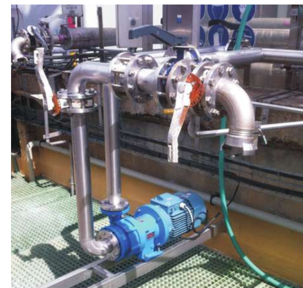
C MAG-PL80 applied for truck unloading of H 2 SO 4 at 96% concentration
